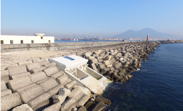
Figure 3 - Breakwater equipped with the OBREC prototype in the port of Naples
