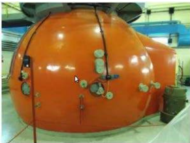
Fig.3: The TAPIRO facility hall.
