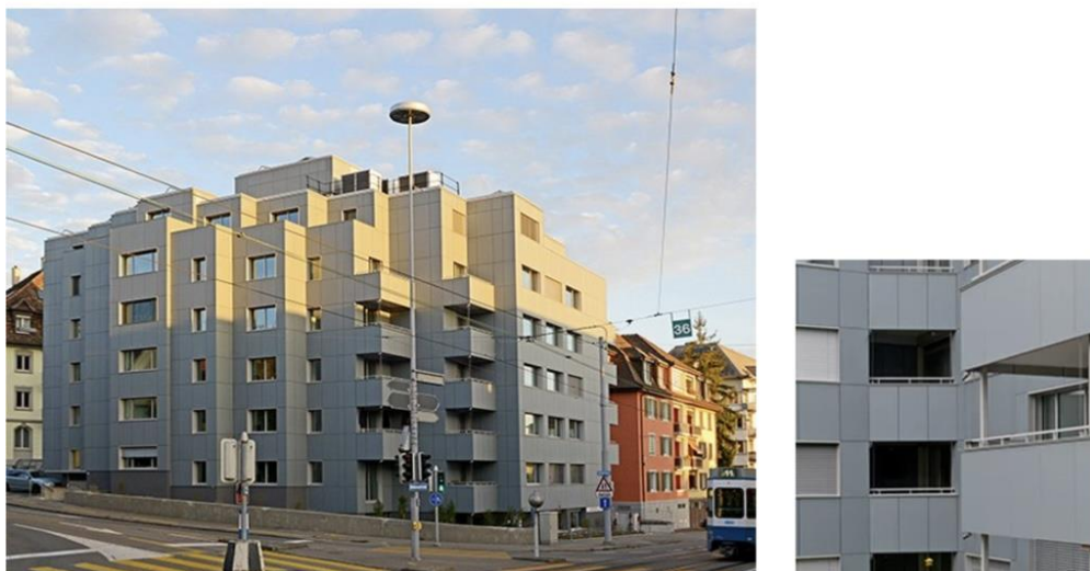
Figure 5. Apartment building on Hofwiesen- and Rothstrasse, renovation and expansion, Zürich (CH), 2016. Design: Viridén + partner. In detail: the facade is composed of a few types (size) rectangular modules showing an opaque, uniform gray surface. Pictures © Viridén + Partner AG, Zürich.
