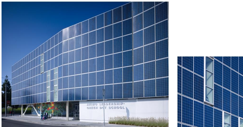
Figure 3. Green Dot Animo Leadership High School, Inglewood, California (USA), 2013. Design: Brooks + Scarpa Architects. On the right: standard (opaque) photovoltaic modules are used. Pictures: © John Linden.
