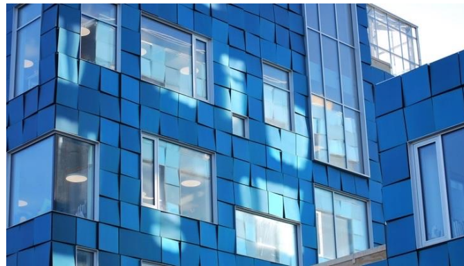
Figure 18. The grain of a pattern depends on the size of the single spatial units, defined by their borders. The border can correspond to a technological component, such as a frame, but also to the simple perception of the condition of not coplanarity of two adjacent spatial units. In the picture, a detail of the facade of the Copenhagen International School, Copenhagen (DK), 2017. Design: C. F. Møller Architect.
