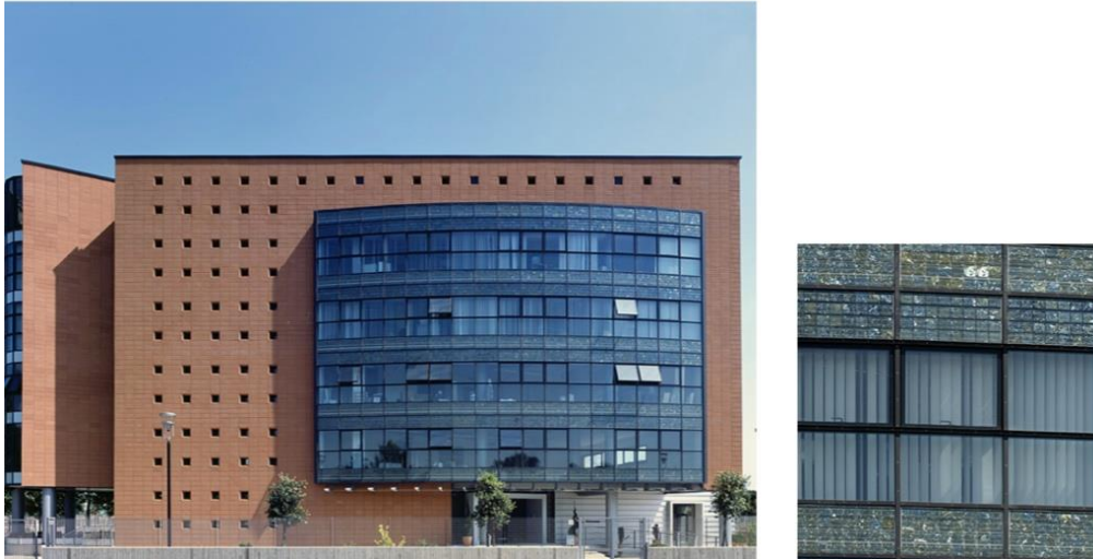
Figure 4. CMB headquarters, Rome, Italy (2006). Design: 3c+t, Capolei Cavalli architetti associati. In the glazed part of the building’s facade glass–glass photovoltaic modules alternate horizontal areas with transparent glass. In detail: the photovoltaic glass–glass modules are semitransparent, because of the distancing of the photovoltaic cells. Pictures courtesy of Fabrizio Capolei.
