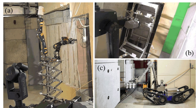
FIG. 9. Three of the main tasks carried out by robots: (a) CERNBot2.0 with double arm configuration cutting cables; (b) Teodor installing the shelf structure on the n_TOF's spallation original target pool; (c) Telex robot installing an intermediate support with six sample containers in the NEAR irradiation station (CERN-PHOTO-202107-085-7) [39].
