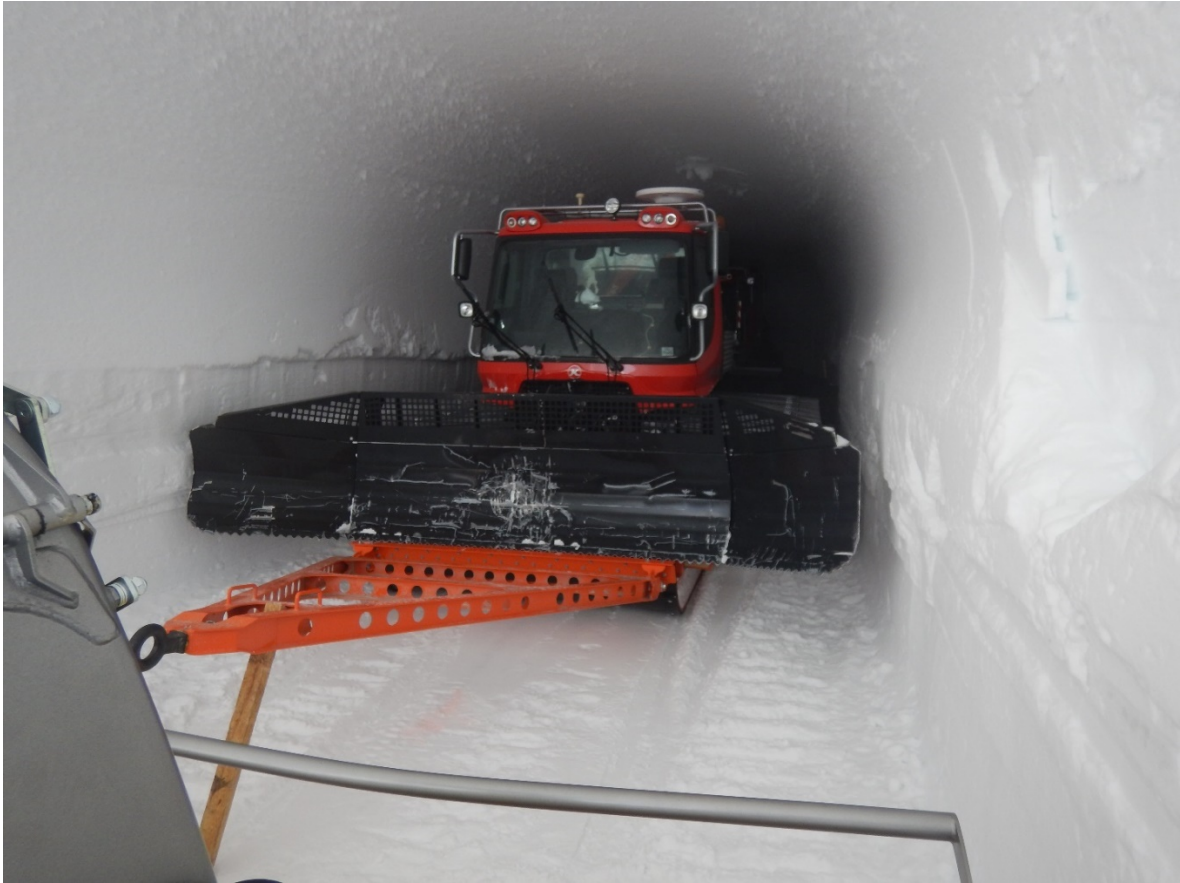
Figure 12. internal of the garage cave at the opening of the door after the winter of 2021. on the roof, the growing of the ice crystals due to the humidity of the air is slightly evident.
