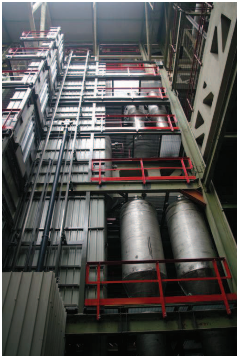
Figure 7 – SPES 3 steel structure
