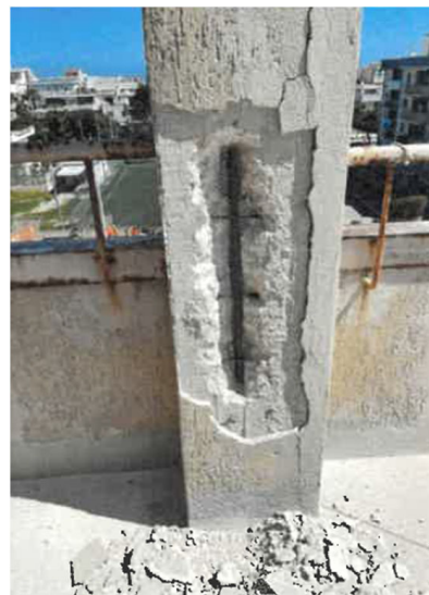
Figure 11. A column rebar before the extraction.
