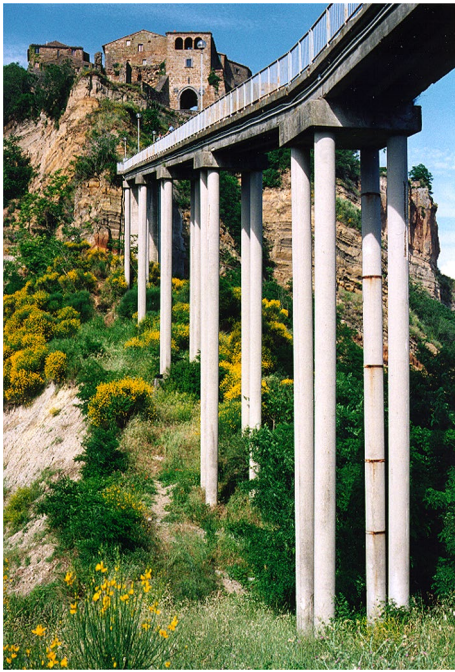
Fig. 7 The tallest part of the viaduct, from piers 1 to pier 5
