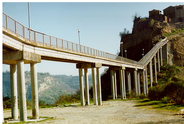
Fig. 2 View of the bridge
