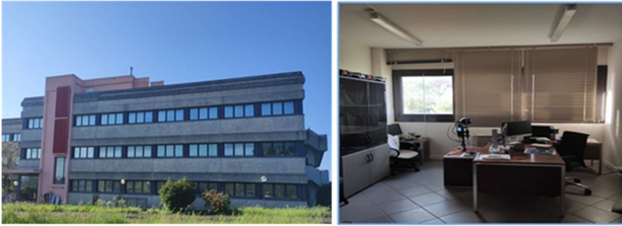
Fig. 1. Case study: building F83, ENEA Casaccia Research Centre in Rome (left) and “typical office room” (right).
