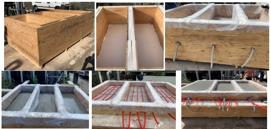
Figure 4. Some phases of the installation of the RTC Box.
