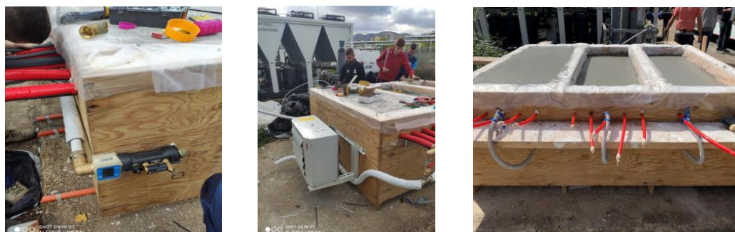
Figure 5. Some phases of the installation of the RTC Box.
