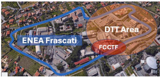
Fig. 1. Aerial view of ENEA Frascati research center including the DTT and the FCCTF areas.
