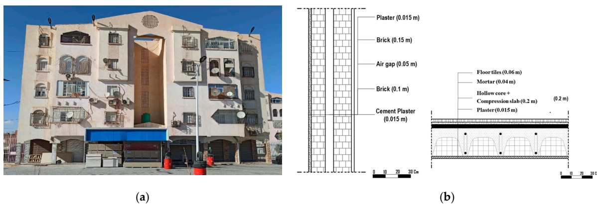
Figure 4. (a) Outdoor façade of the first case study; (b) external walls and roof Components (Source: Authors, 2025).
