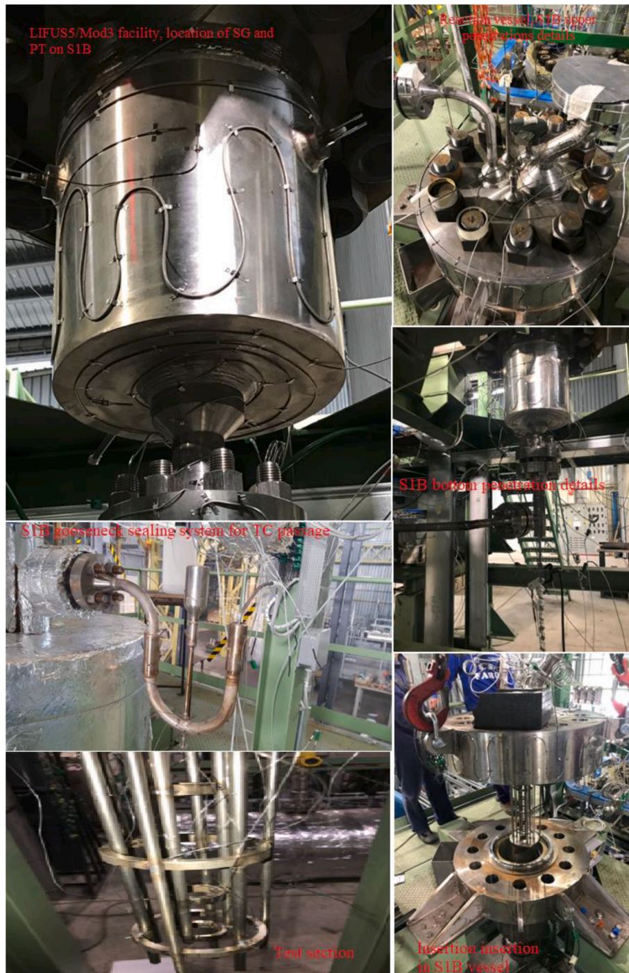
Fig. 4. Real pictures of LIFUS5/Mod3 facility during commissioning phase.
