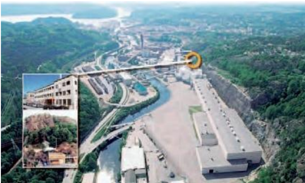
Fig. 1. Site area of the BHWR in Halden.
