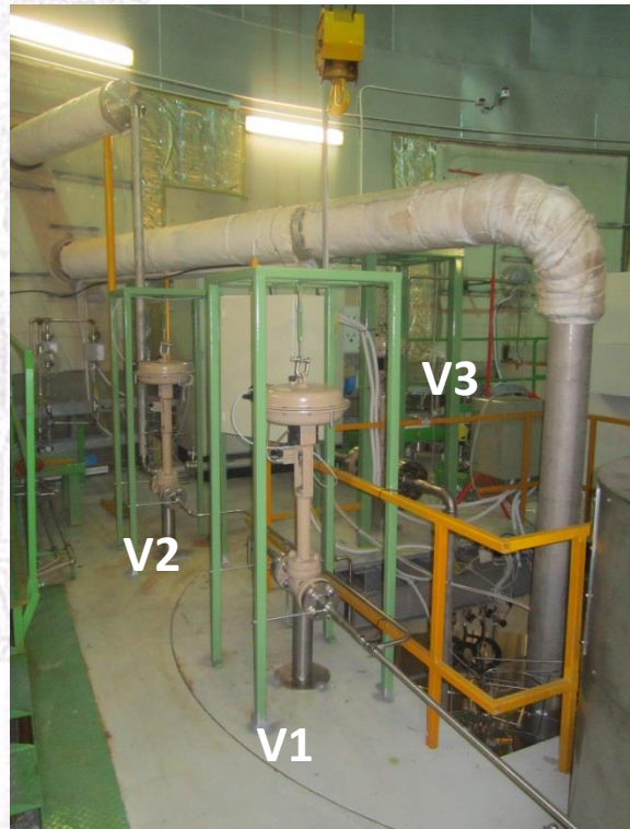
V1 isolation valve V2 bypass valve V3 regulation valve
