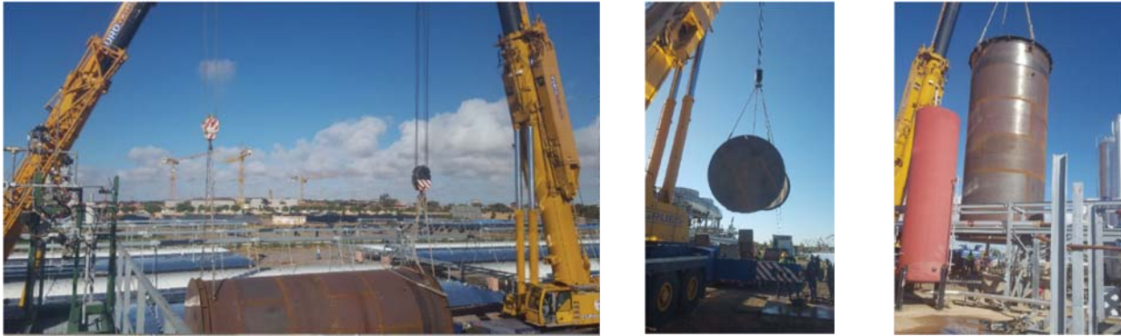
FIGURE 2. Some steps of the installation of the TES tank.
