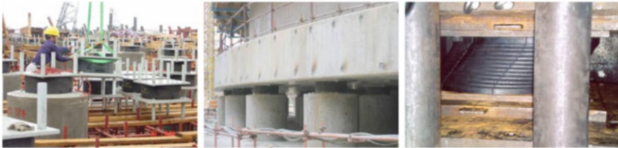
Fig. 14.32 Left : one of the two seismically isolated LNG tanks in the Guangdong Province (Southern China) during construction (each of them was isolated by means of 360 HDRBs). At the centre : some of the isolators after their installation. Right : a HDRB during acceptance tests
