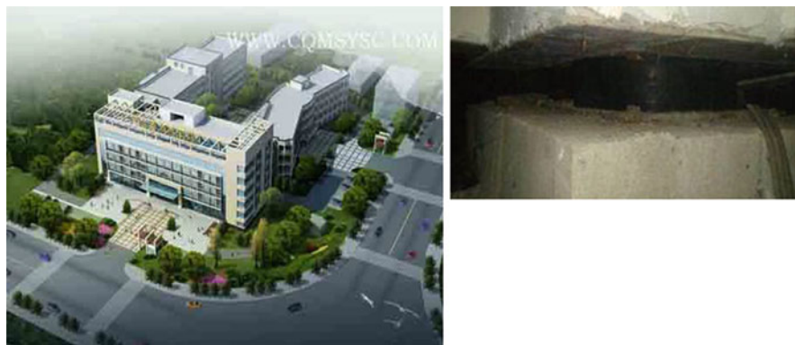
Fig. 14.9 View of the Lushan county hospital (China), before the earthquake of April 20, 2013 (Zhou et al. 2013)
