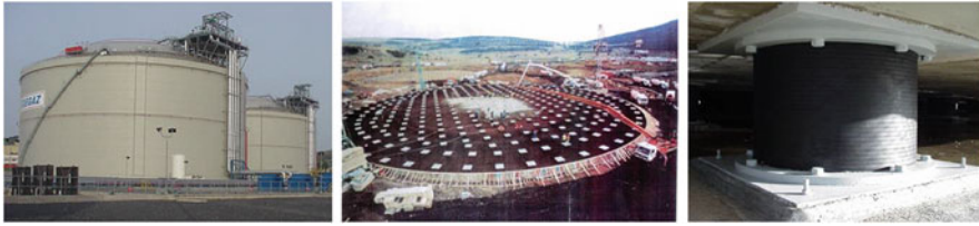
Fig. 14.31 Left : one of the two LNG tanks of Egegaz in Aliaga (Turkey), which were seismically isolated using 112 LRBs and 241 LDRBs. At the centre : view of the isolators during construction. Right : an installed LRB
