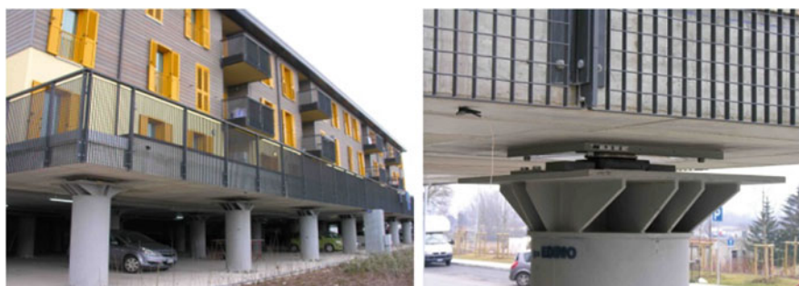
Fig. 14.20 Left : one of the 184 pre-fabricated houses (wood, or r.c., or steel structures) erected in L'Aquila to host up to 17,000 residents who remained homeless after the 2009 Abruzzo earthquake. Right : detail of one of the 40 CSS devices, manufactured in Italy, which have been installed at the top of columns (made of steel or r.c.) to isolate the supporting slabs of such houses
