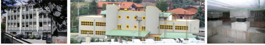
Fig. 14.29 Left : the Romita High School in Campobasso (Italy), in 2003 (when it hosted 1,300 students), before the demolition of its two most unsafe A and B blocks and reconstruction of block A with SI (see Fig. 14.18). At the centre and right : the new school of Marzabotto (Bologna, Italy), former seismic zone 3), which was seismically isolated (with the collaboration of ENEA) by means of 28 HDRBs and 14 SDs, with 500 mm diameters; it is the first seismically isolated school in Northern Italy, which was certified as safe by A. Martelli in September 2010
