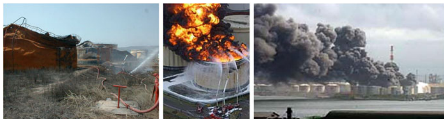
Fig. 14.27 Left : rupture of a storage tank in the Yarimca Refinery (Turkey), owned by Tupras, during the Izmit earthquake of August 17, 1999 ( M_W = 7.4 ), which caused 17,000 victims. At the centre: initial fire of one the two tanks (the first containing crude oil, the second naphtha) of the Tomakomai City petrochemical installation (Japan), caused by the two main shocks of the Off Tokachi earthquake of September 26 and 28, 2003 ( M = 8.0 and M = 7.1 ), with epicenters at 220 km from the plants. Right : propagation of the fire in the Tomakomai City petrochemical installation, during the aforesaid quake, with the consequent damage of 45 tanks (30 severely, 29 with leakage) of the 105 present
