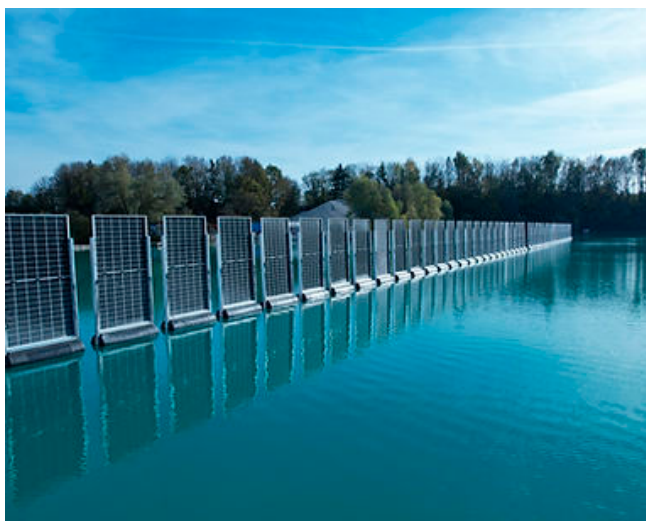
Figure 5. Bifacial vertical floating PV systems proposed by Sinn Power GmbH. SINN Power image. Adapted from [31].
