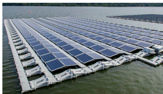
Figure 1. Floating pontoon with walkway—© 1996–2025 MDPI image. Adapted from [23].
