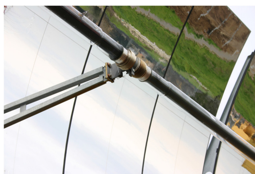
Figure 8. A view of the receiver tube brackets.
